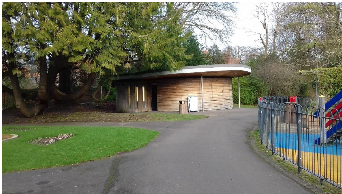
Borough Gardens Kiosk and Toilets
